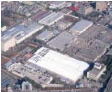
NSK Fujisawa Plant
