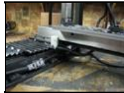
X Axis Limit Switch Covered 2
